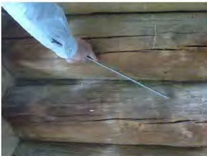
Fixing/ reinforcement with screws d=8\text{mm} in the walls.
